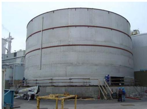
Figure 1. A white liquor tank made of LDX 2101 for the cellulose industry.
