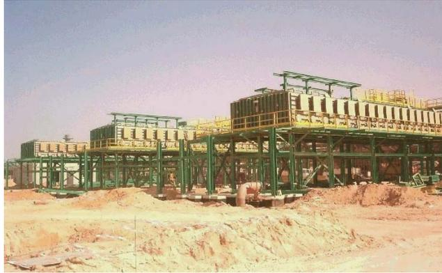
Figure 3. Melittah MSF recycling plant with solid duplex stainless steel evaporator shells.
