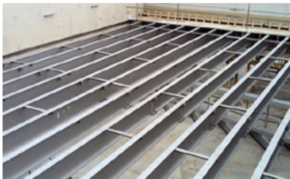
Beckton Desalination Plant Courtesy of Millstock Stainless
